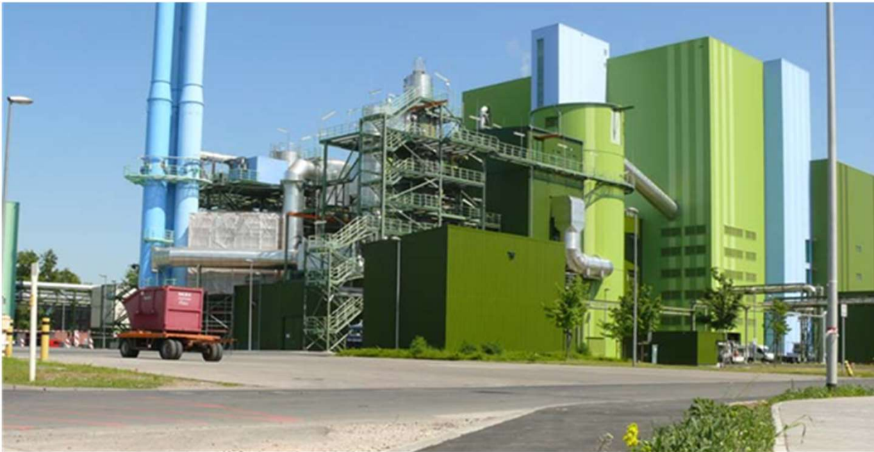
Waste CHP Station Mainz, Mainz, Germany
